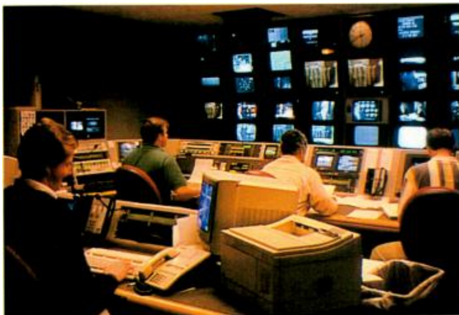
The networked control room will allow WXYZ staff to direct the on-air playback of both HD and multichannel using Omnibus networking and Profile servers.
